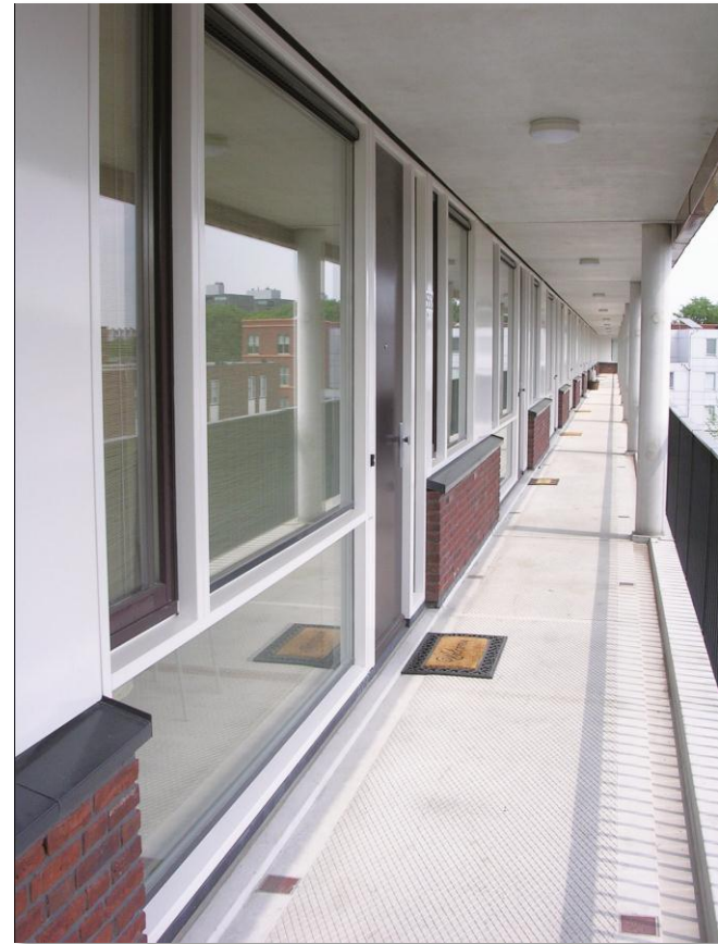
Finger-jointed acetylated wood used to manufacture windows
